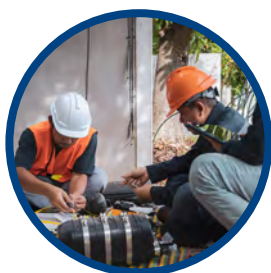
Fiber Installation Verification
